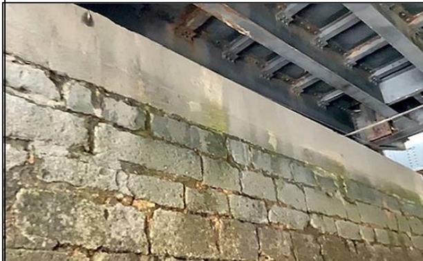
Outer Bridge showing concrete pillow block along top of masonry side wall of canal. This replaced several removed courses of stonework.
