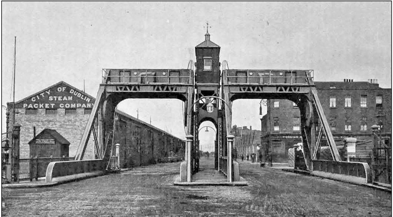
**1913** View from west towards City end showing both bridges open for road traffic. The motors which powered each of the bridges are visible half-way along each gantry in front of the overhead counterweights. (*Griffith 1913*)
