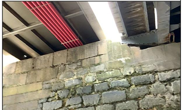
Looking W showing one of the 2019 spans carried over the top of the canal's side wall. By contrast, the end of the Outer Bridge (*at right*) is let into its top.
