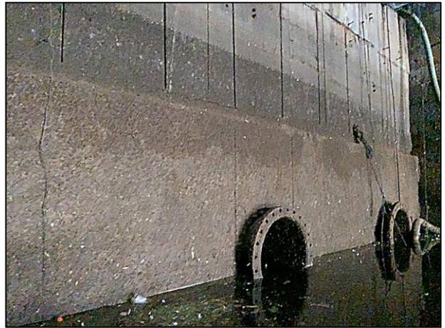
Concrete wall across lock chamber, with drainage pipes along bottom.
