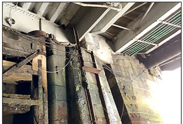
Lock gate on east side. Note the vertical slot at right for timber baulks to cut the channel off from the river.
