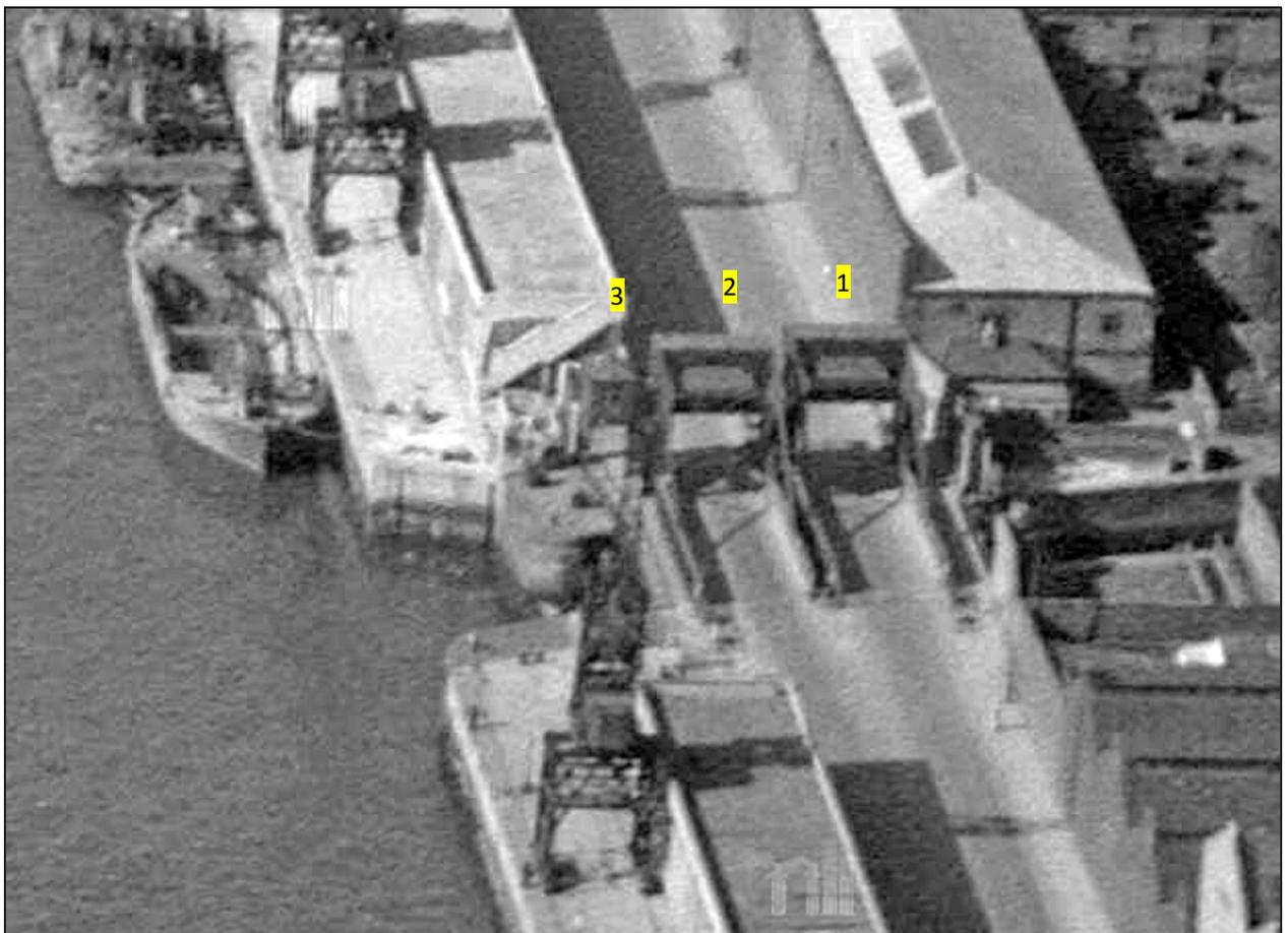
Fig 6.8 Aerial views of Scherzer bridges over entrance to George's Dock, from east. Top: 1949 view (*Britain from Above*, XAW027127). Bottom: 1955 view (*National Library Ireland, Morgan Aerial Photographic Collection*). Key: 1 - Inner Bridge, 2 - Outer Bridge, 3 - Overhead control cabin.
