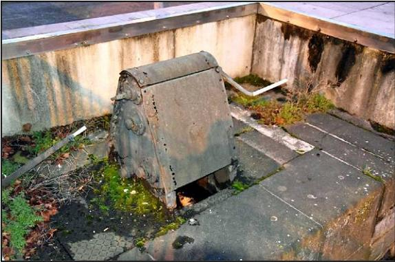
Fig 3.9 One of the two winches used to open and close the repositioned timber lock gates underneath the Inner Bridge.
