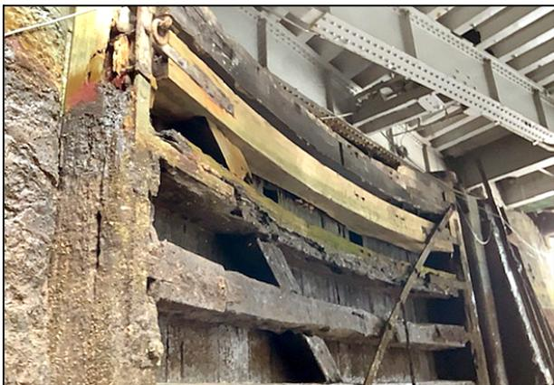
Curved timber lock gate on west side of channel underneath Outer Bridge.
