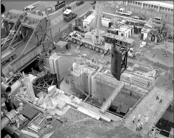
Fig 3.10 Installation of new sea lock gates, 2008 (Delaney & Bath 2010, p.306).
